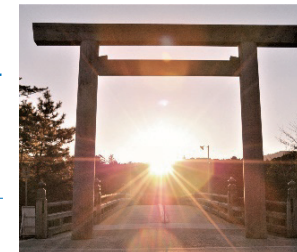
Ise Grand Shrine (Large Torii gate at Uji Bridge)
