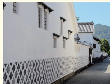
Traditional white walls and white plaster namako walls of the Hagi castle town
